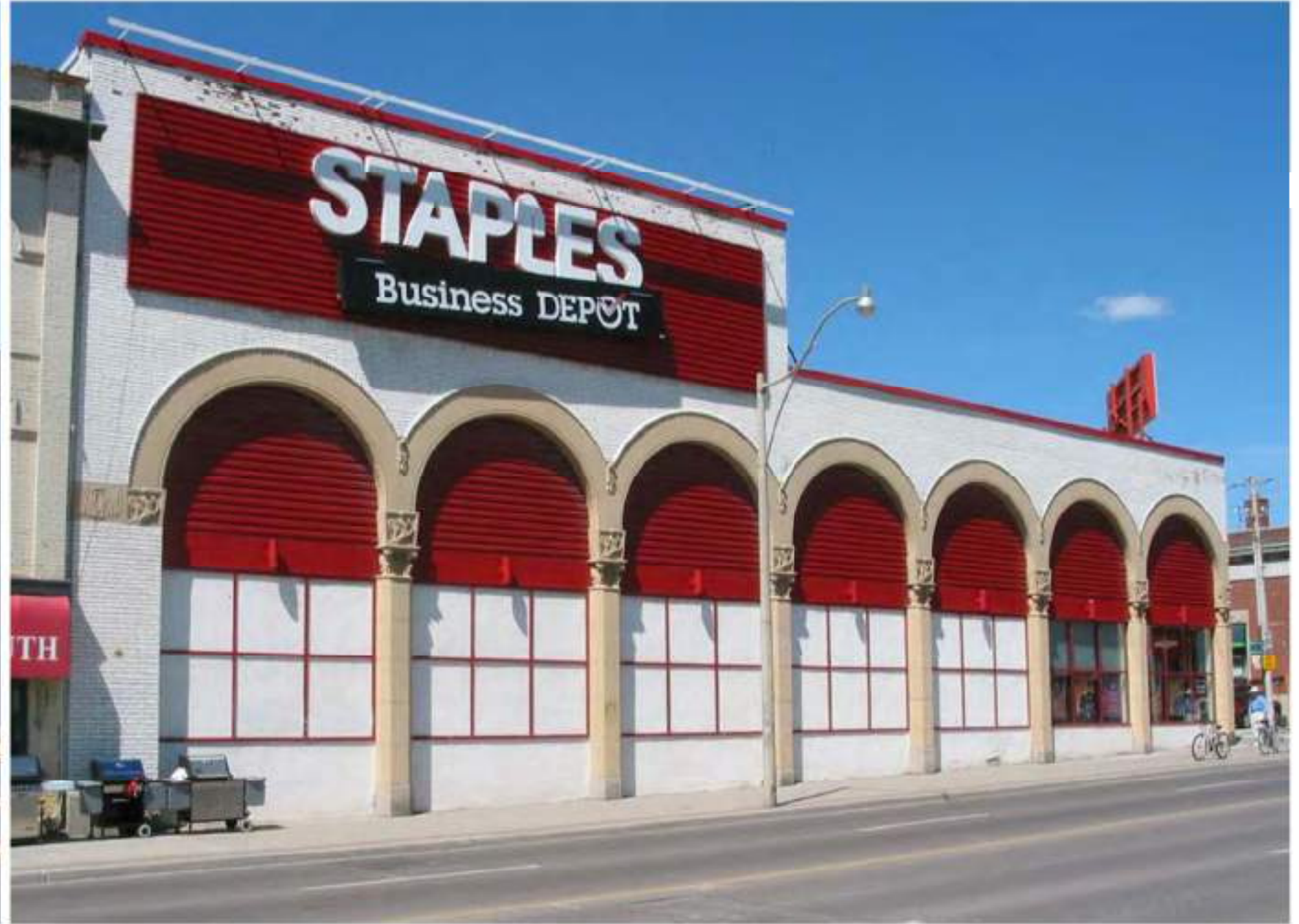
WEST FACADE ON YONGE STREET
